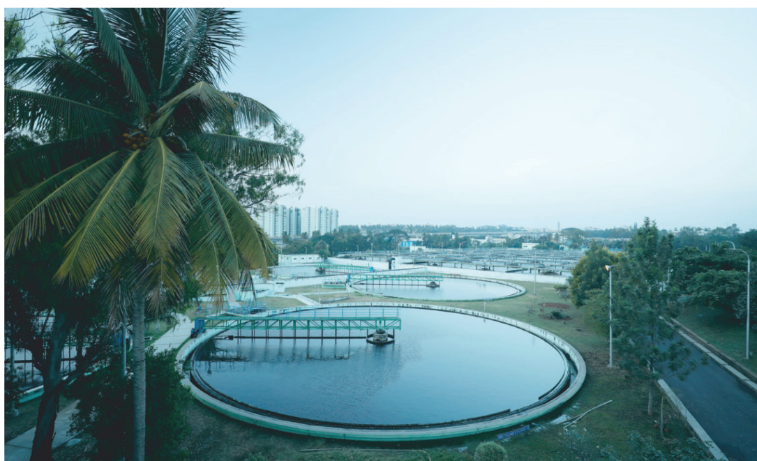
Fig. 20.8. Sewage water treatment plant
